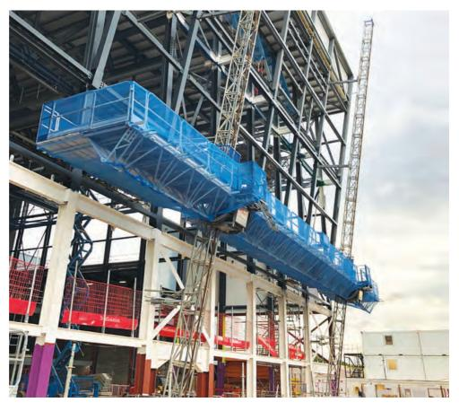
When it came to installing cladding on the new £83m, 26,000 sq m **International Convention Centre** (ICC) outside Newport in Wales, subcontractor Massey Cladding, working with main contractor Sisk, needed a mast-climbing work platform (MCWP) solution to ensure that work could be carried out safely.
