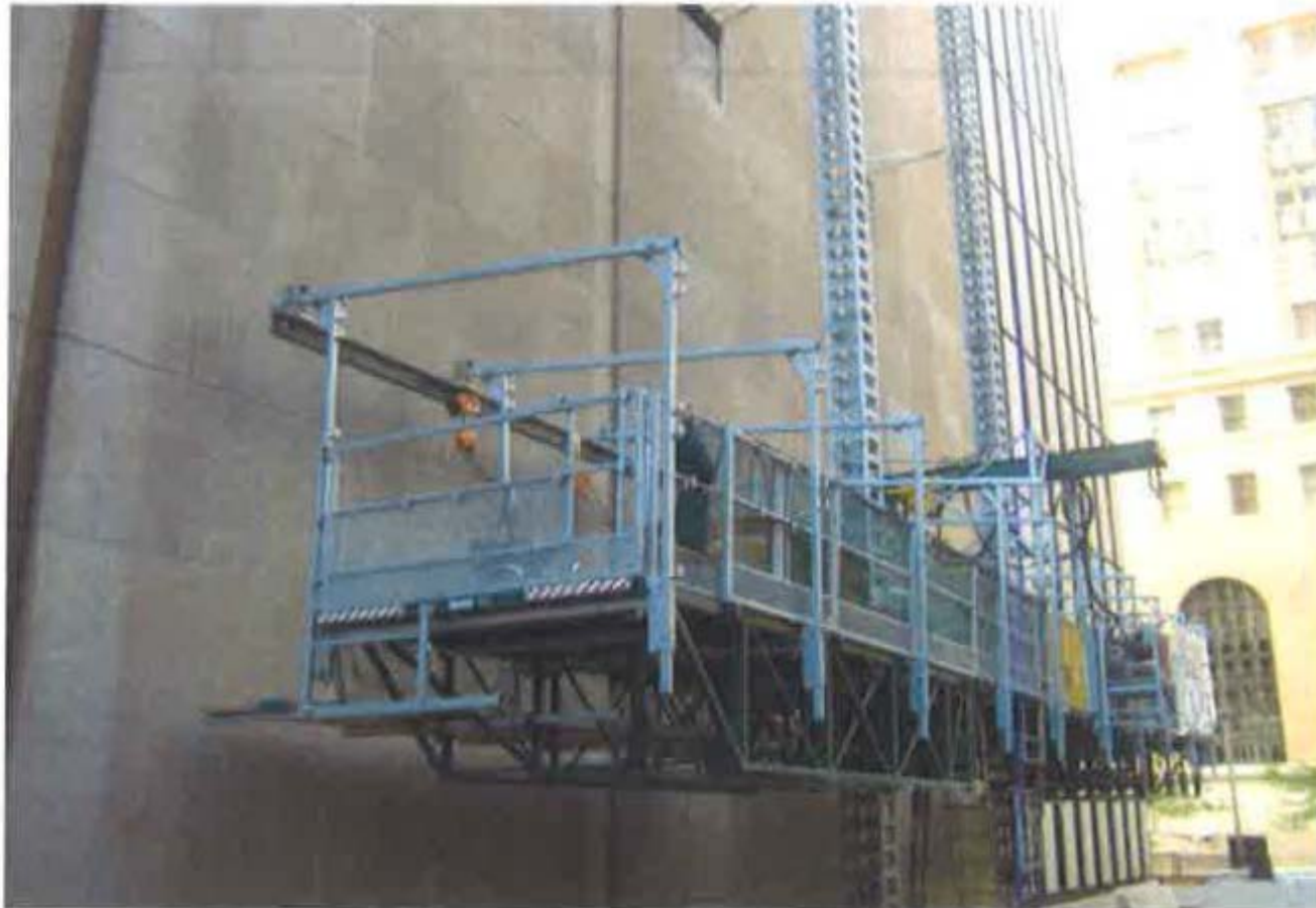
Photo 9: Mast Climber with Non-Swinging Mounted Monorail Hoist
