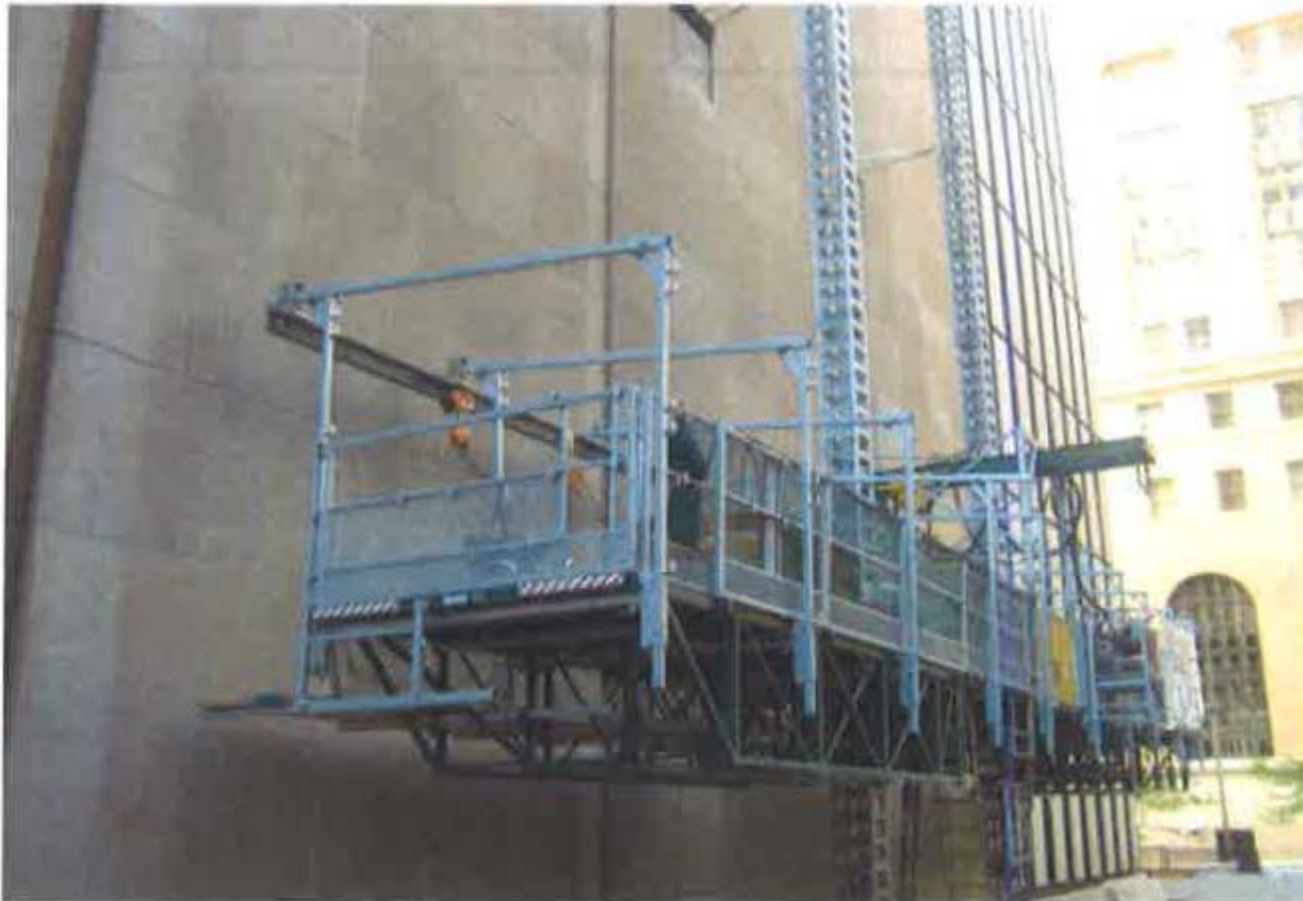
Photo 9: Mast Climber with Non-Swinging Mounted Monorail Hoist
