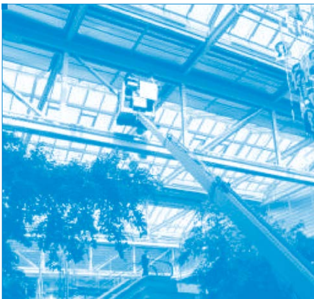
Example 6: Cleaning glass atria and roofs from the inside using a suspended seat (rope access and positioning techniques)
