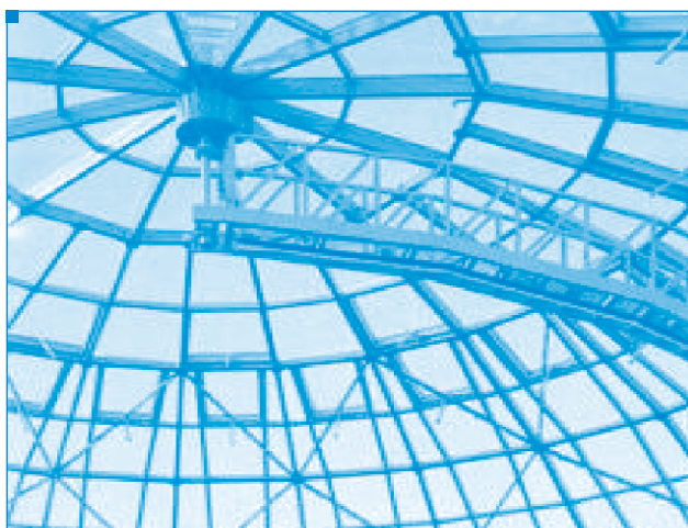
Example 2: Cleaning glass atria and roofs from the inside using a tower scaffold
